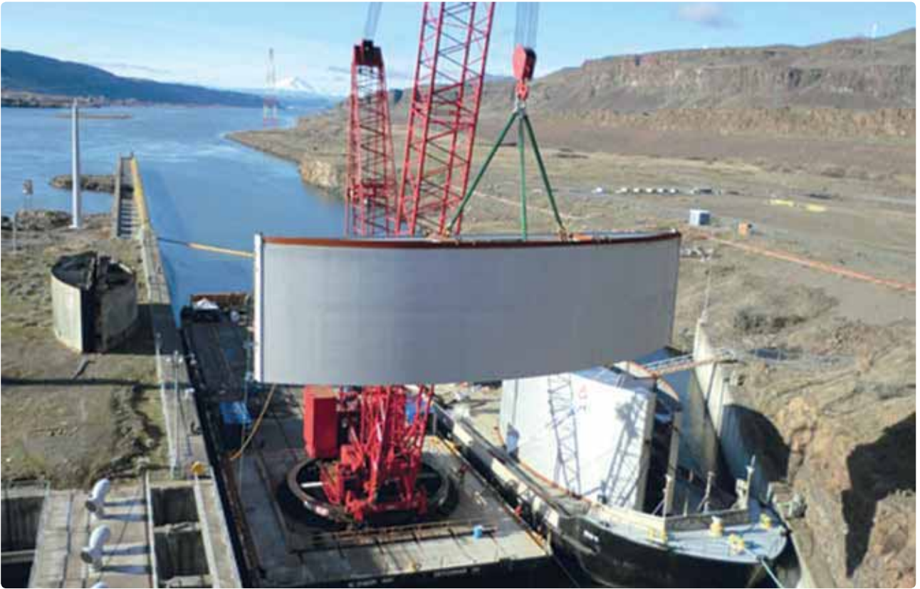
Twin-Path® slings lift a 275 tonne floodgate.
