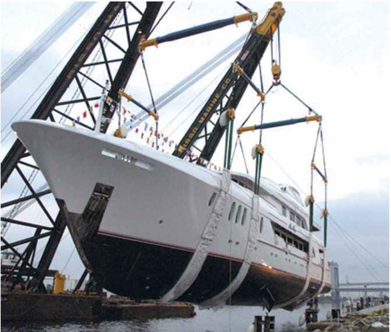
672 tonne super yacht lift using TwinPath® Slings and CornerMax® Sleeving.
